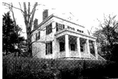
This c1836 Greek Revival building at 92 Harrison Street is one of the many architectural beauties in Stapleton. SIAS Architectural Survey.
